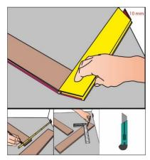
Measure and cut the end panels to size using a fine-toothed saw. Finish the first row with the cut end panels. Make sure that you leave a gap of 10 mm to each wall.
